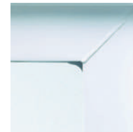
Vinyl sash corner seam
